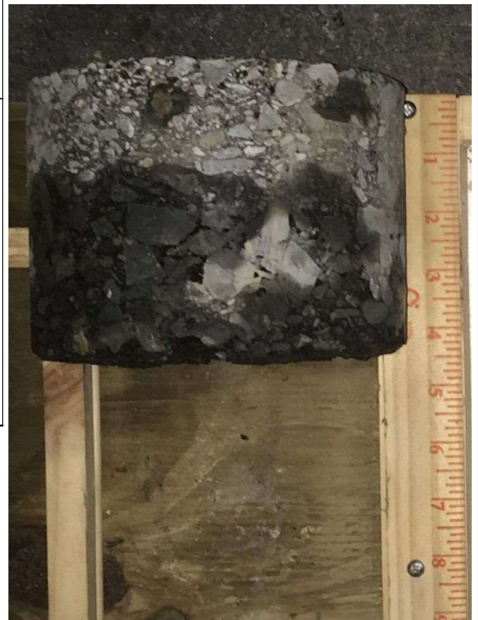
Bottom of Pavement Core 1.7' below ground surface.
