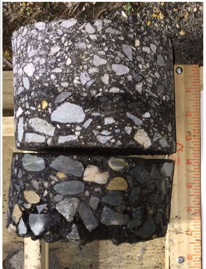
Bottom of Pavement Core 1.8' below ground surface.
