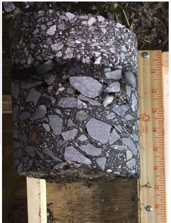
Bottom of Pavement Core 1.6' below ground surface.
